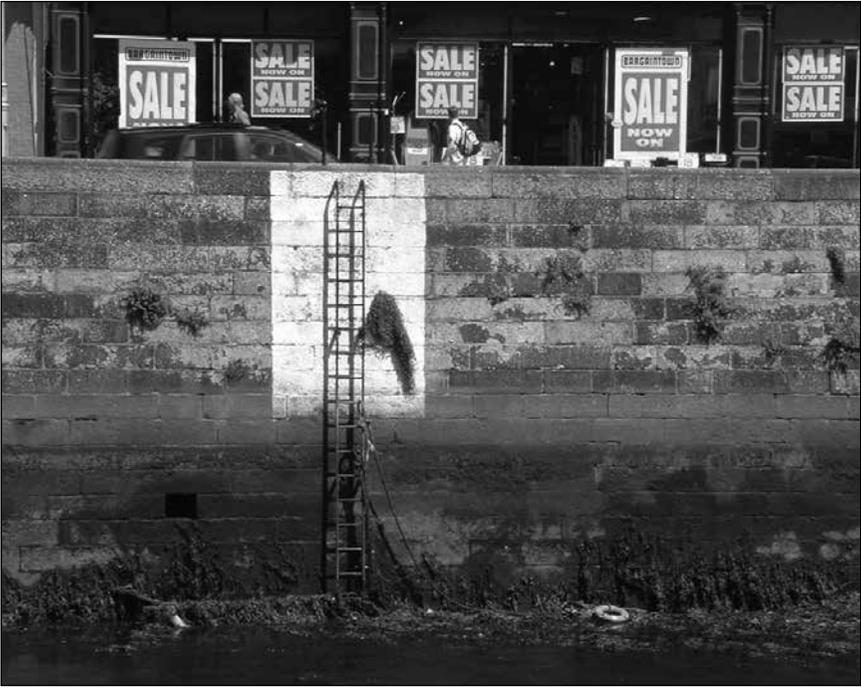
**Figure 4** –Wall behind a ladder in the River Liffey, Dublin, painted white to highlight an exit place.
