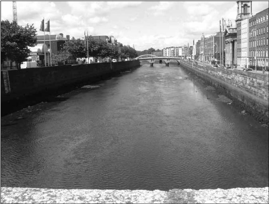
**Figure 2** – High, steep stone walls used to contain the River Liffey, Dublin.
