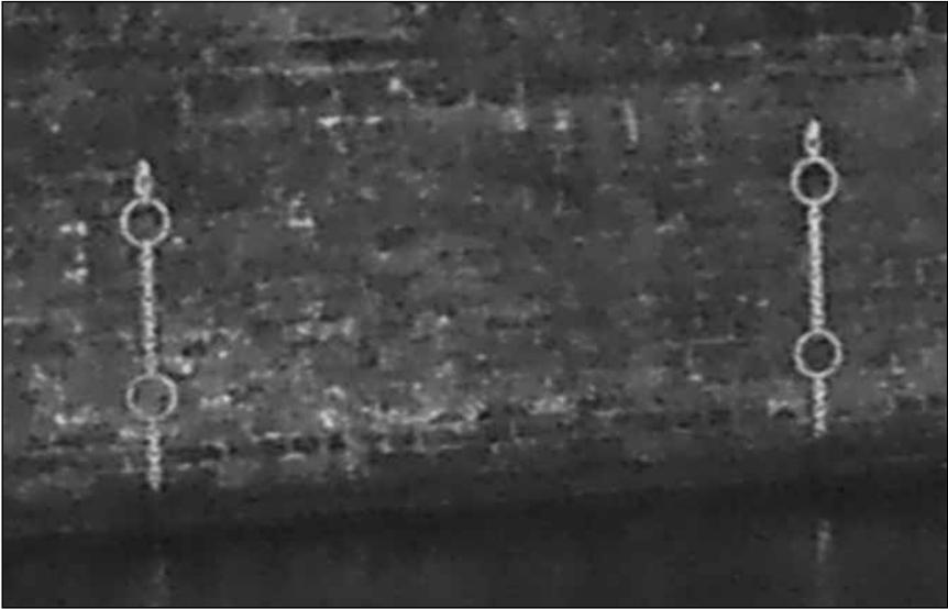
**Figure 5** – Victorian grab chains in Liverpool Docks (UK) to enable persons to climb out of the water.
