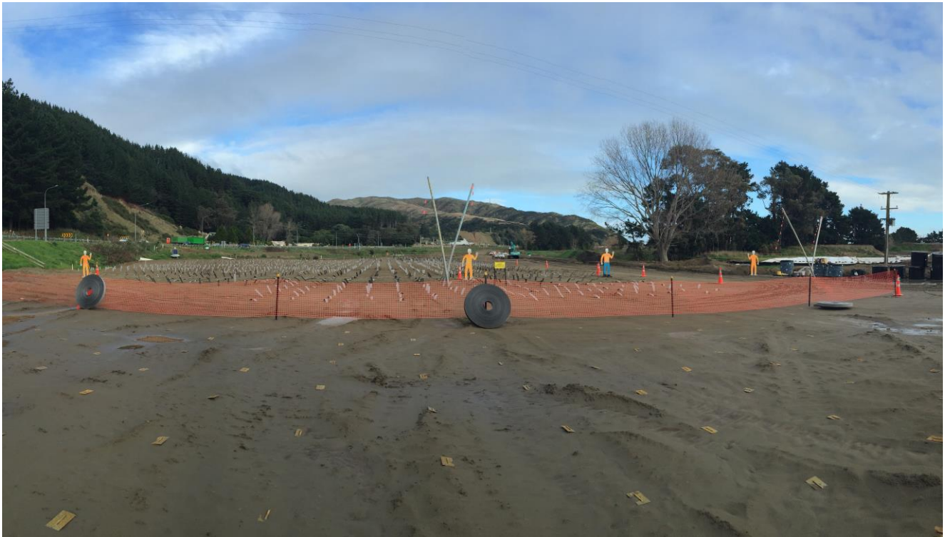
Image: Life-size plywood cut-out construction workers guard sensitive equipment during fill operations to support construction of the Transmission Gully Motorway just north of Paekakariki.
