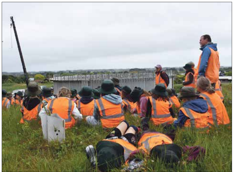
Students of Waitohu School watch construction of the Ōtaki reservoir at the top of Te Manuao Road. Photo Ōtaki Today
