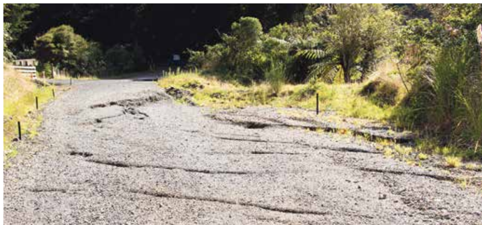
NO GO: Cracks and slumping at Blue Bluff have closed the road.
