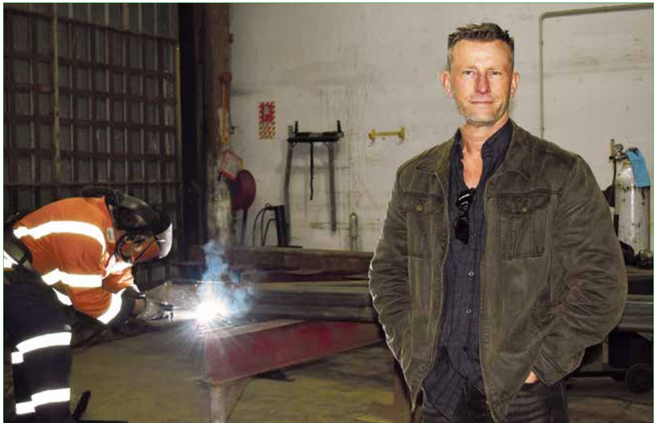
Dean Roberts at Riverbank Engineering on Riverbank Road. Simon Haines is behind welding one of the brackets for the Ōtaki River bridge shared path. Photos Ōtaki Today
