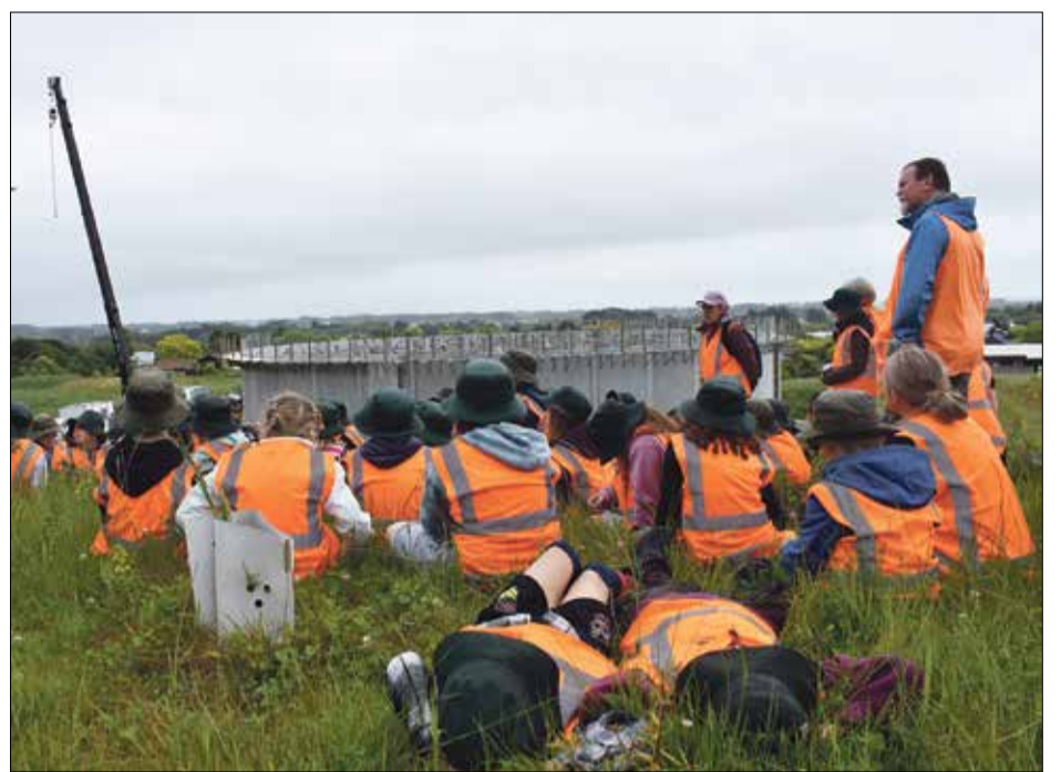
Students of Waitohu School watch construction of the Ōtaki reservoir at the top of Te Manuao Road. Photo Ōtaki Today
