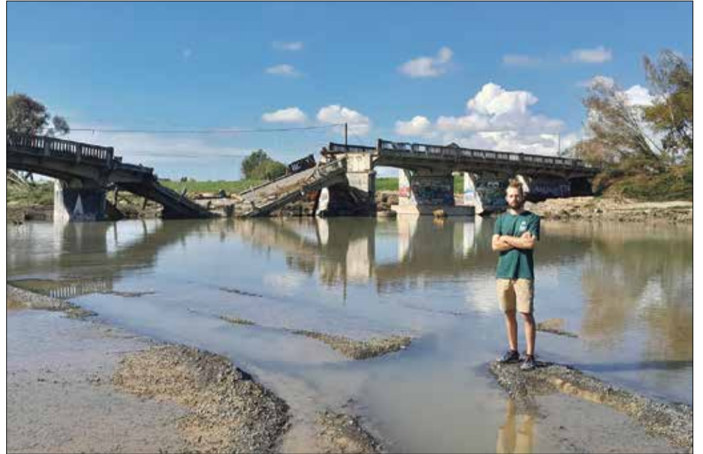
Tom Kay at Redclyffe Bridge in Hawke's Bay after Cyclone Gabrielle.
