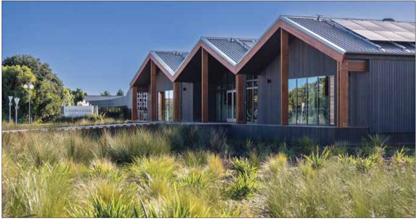
Part of the wetland area Pritchard Civil helped to develop near Tasman Road.
