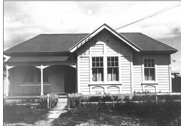
In 1911 the house at 3 Iti Street was built as Ōtaki's police station with the residence attached.
