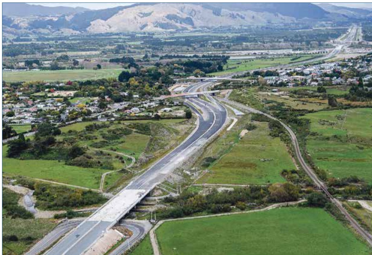
ROADWAY: A view of the expressway from the northern end with the new Waitohu Stream bridge in the foreground.
