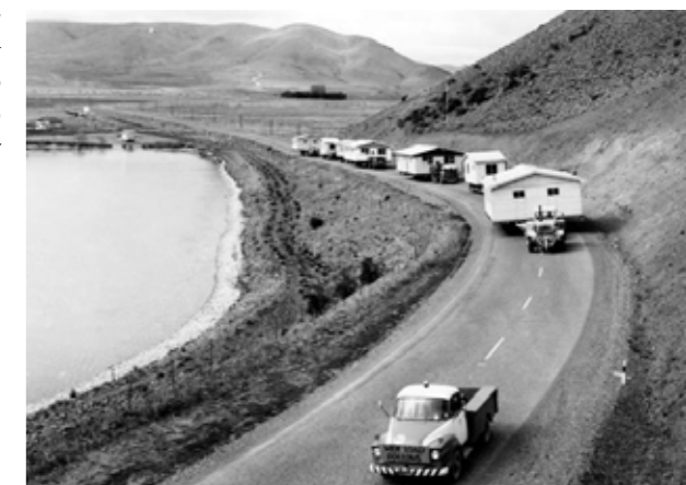
Right: Oamaru company De Geest delivering homes to Twizel, along some 150 km of windy roads.
