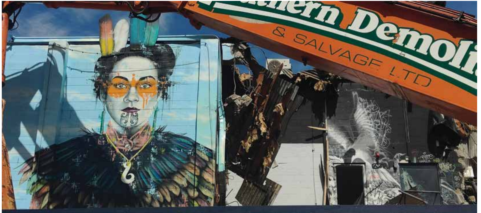
↑ Fin Dac's Kaitiaki is demolished as the Hereford Street YMCA building prepares for rebuilding. A mural produced in tribute to Palestinian activist Mahsa Amini by Kophie Sua-Hulsbosch - produced in collaboration with the Kia Ora Academy
